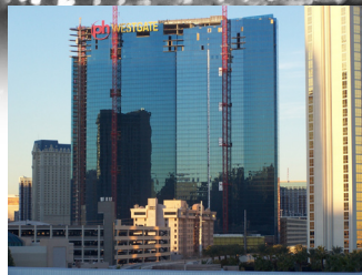
Planet Hollywood Towers $1.2 Billion
